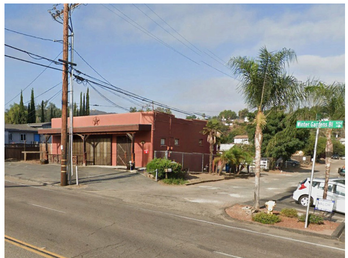
Missing sidewalks along Winter Gardens Boulevard near Riverview Elementary School
