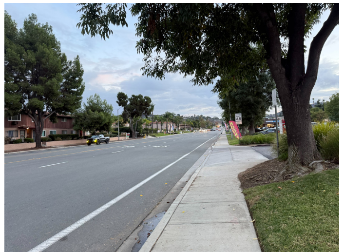
Four-lane undivided roadway with a two-way left-turn lane along Winter Gardens Boulevard
